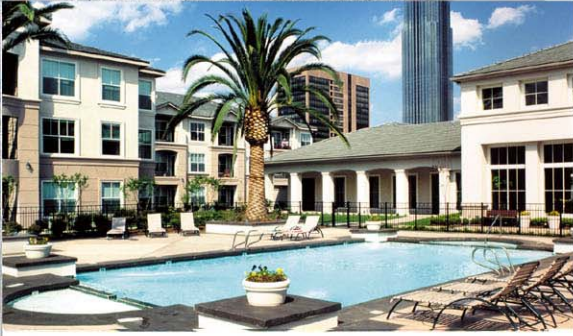
The Terrace at Clear Lake for Metro National Corporation
