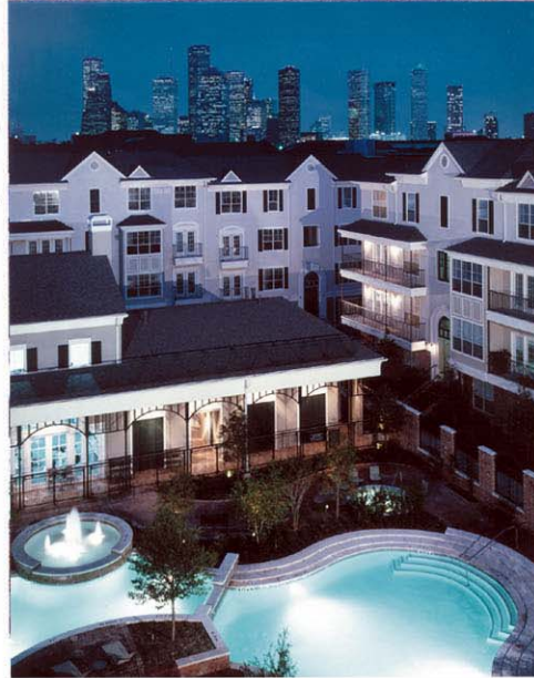
The Quarters at Memorial for McCaslin Development
